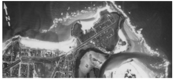
Point Danger and the Tweed River Entrance in 1935, before the Tweed River training walls were extended.
